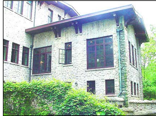
(This is what it looked like outside of the generator room)
